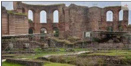
Work began on the Imperial Baths before 300 AD, at the command of Co-emperor Constantius Chlorus (293-306) in Trier, Germany. (Steve ... Read More
