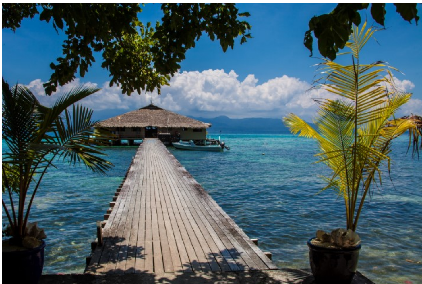
The 100-foot-long pier at Fat Boys Resort connects the Lodge, built on stilts over deep water, with a half-bungalows on shore. The lodge location — the bar, dining room, lounge and kitchen — protects the shoreline water coral and provides a boat dock. PHOTO COURTESY OF STEVE HAGGERTY@COLORWORLD.
